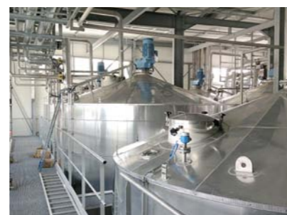
Tankfarm | Tank farm
