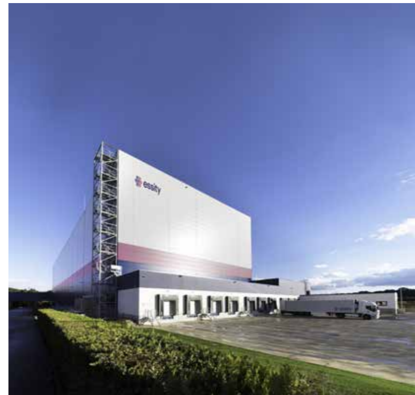
GU-Projekt Hochregallager, Kompetenzzentrum ECE-LOG General contractor project high-bay warehouse, ECE-LOG competence center
