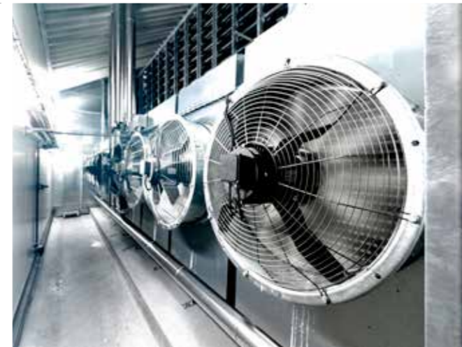
Schockfrostanlage (Luftkühler) Shock freezing system (air cooler)
